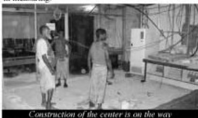
Construction of the center is on the way
