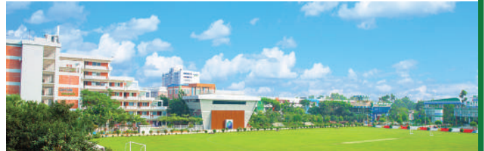
Partial view of the Green Campus
